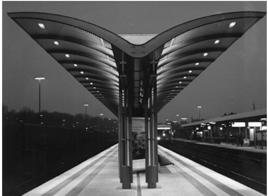
DB AG Platform Designed by von Gerkan of Marg & Partners, Winner of 1996 Brunel Awards
