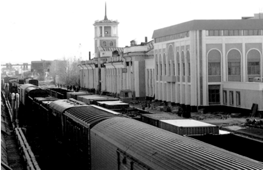
Newly-constructed station building in Lake Baykal region, Siberia. The project was undertaken by Harbin Railway Bureau's International Economic and Engineering Cooperation Company. (CR)
