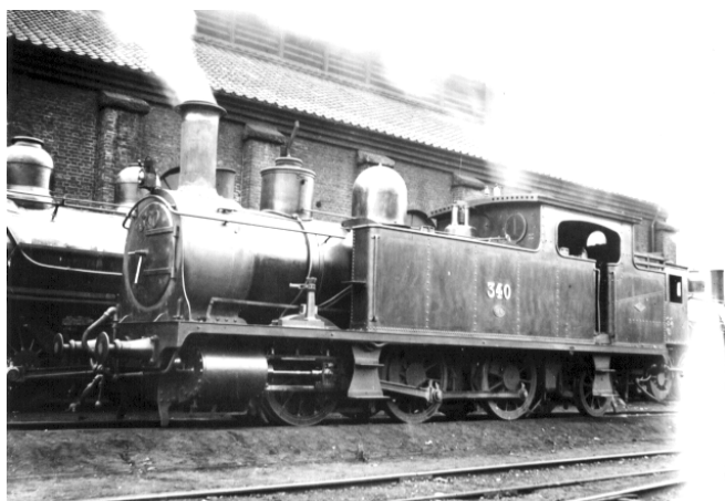
■ Freight locomotive Class 2120. First built as 2100 by Dubs & Co, Glasgow, but much copied by German, American and other British builders around Russo-Japanese War (Transportation Museum)
