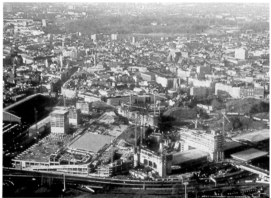
■ Lille-Europe Station under Construction
