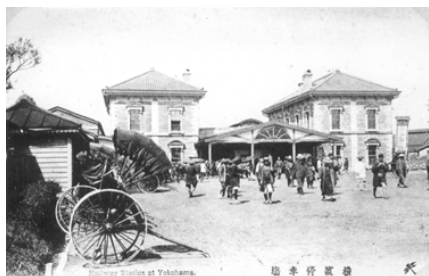
■ Yokohama Station (Transportation Museum)
