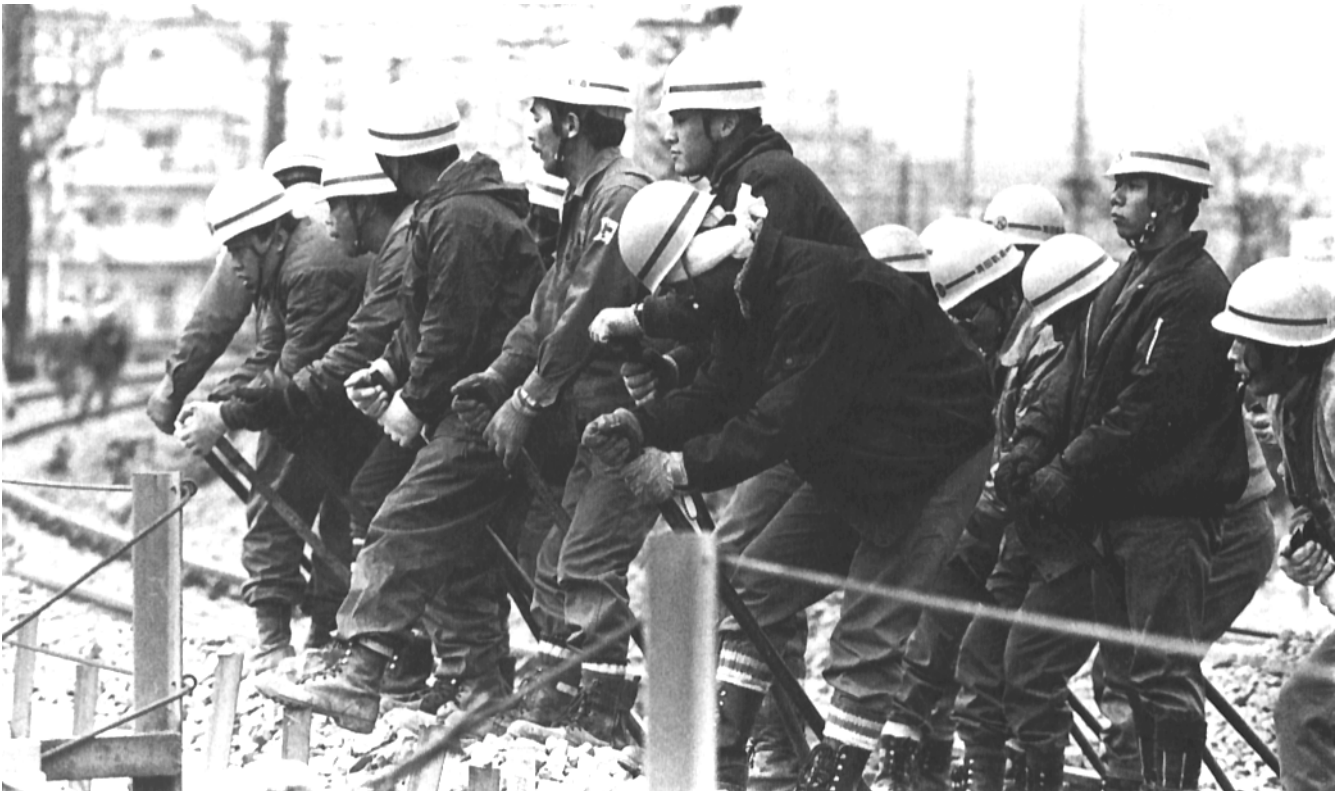
■ Lifting Track on Hanshin Electric Railway
