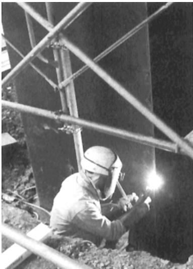
■ Strengthening RC Pillar of Shinkansen Viaduct with Steel Sheathing (Transportation News)
