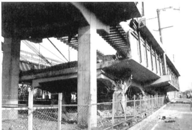
■ Collapsed Sanyo Shinkansen Viaduct
