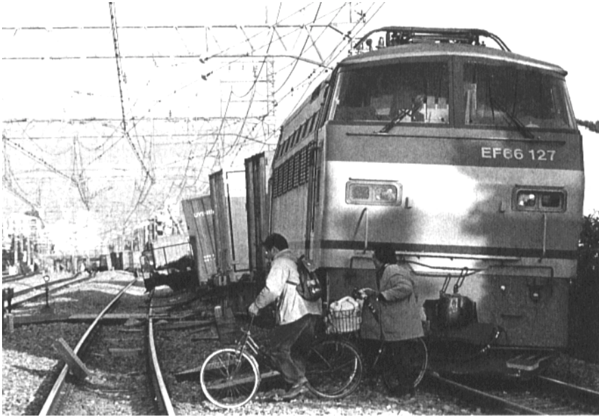
■ Freight Train Derailed in Great Hanshin Earthquake
