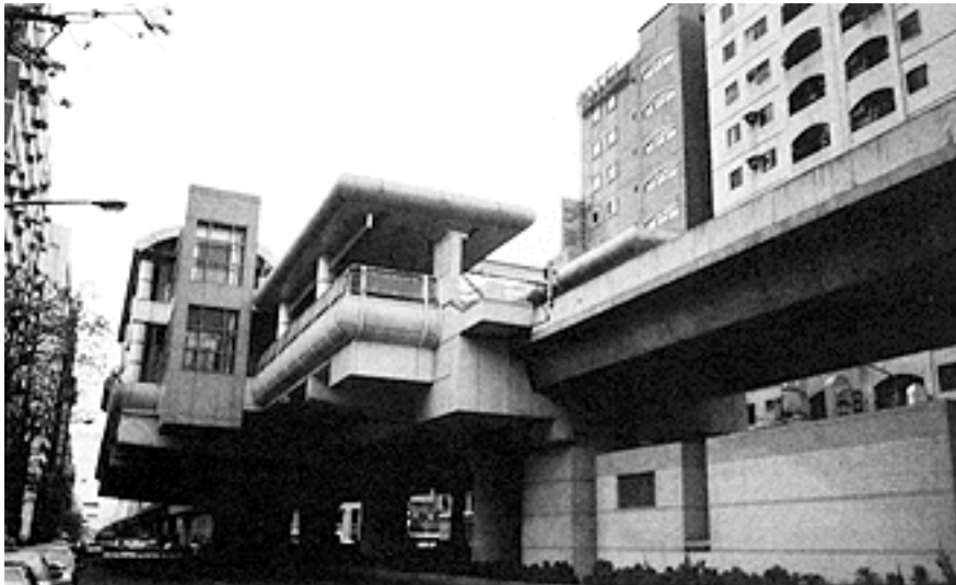
Photo 7 Elevated Structure for Medium-scale Guided Transit in Taipei City - Mucha Line - (Author)
