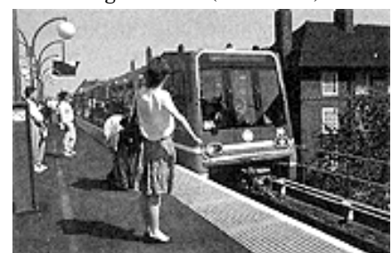
■ Unmanned light rail transit in London Docklands
