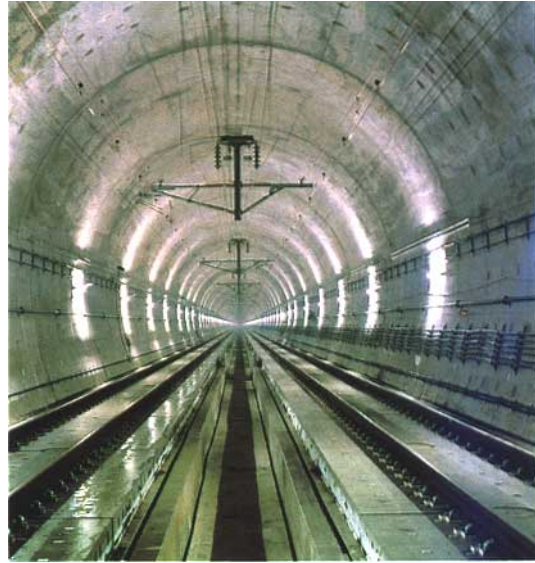
Courtesy: Japan Railway Construction Public Corporation
