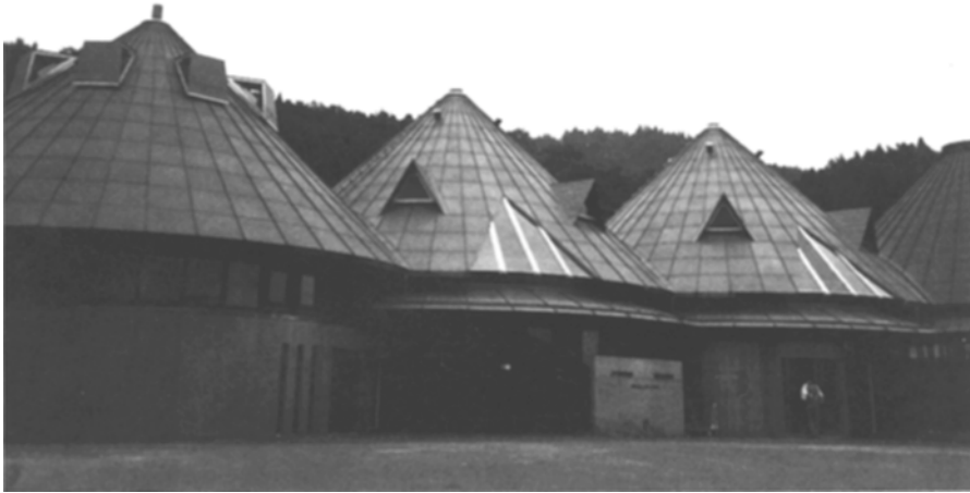
The new Iwaki-Hanawa station was financed both by JR East and the local municipality. It houses a library and a fine-art gallery for local residents.
