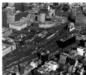
■ Tokyo Station covers approx. 150,000 m 2 of space
